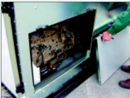
Four access doors swing open and/or lift off
